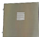
1 Ceiling Air Duct
