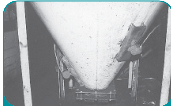
Two Syntron® model TB-320 Pneumatic Turbine Vibrators mounted on a batch hopper.
